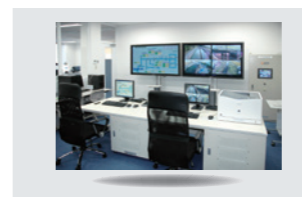
Integrated monitoring and control system
